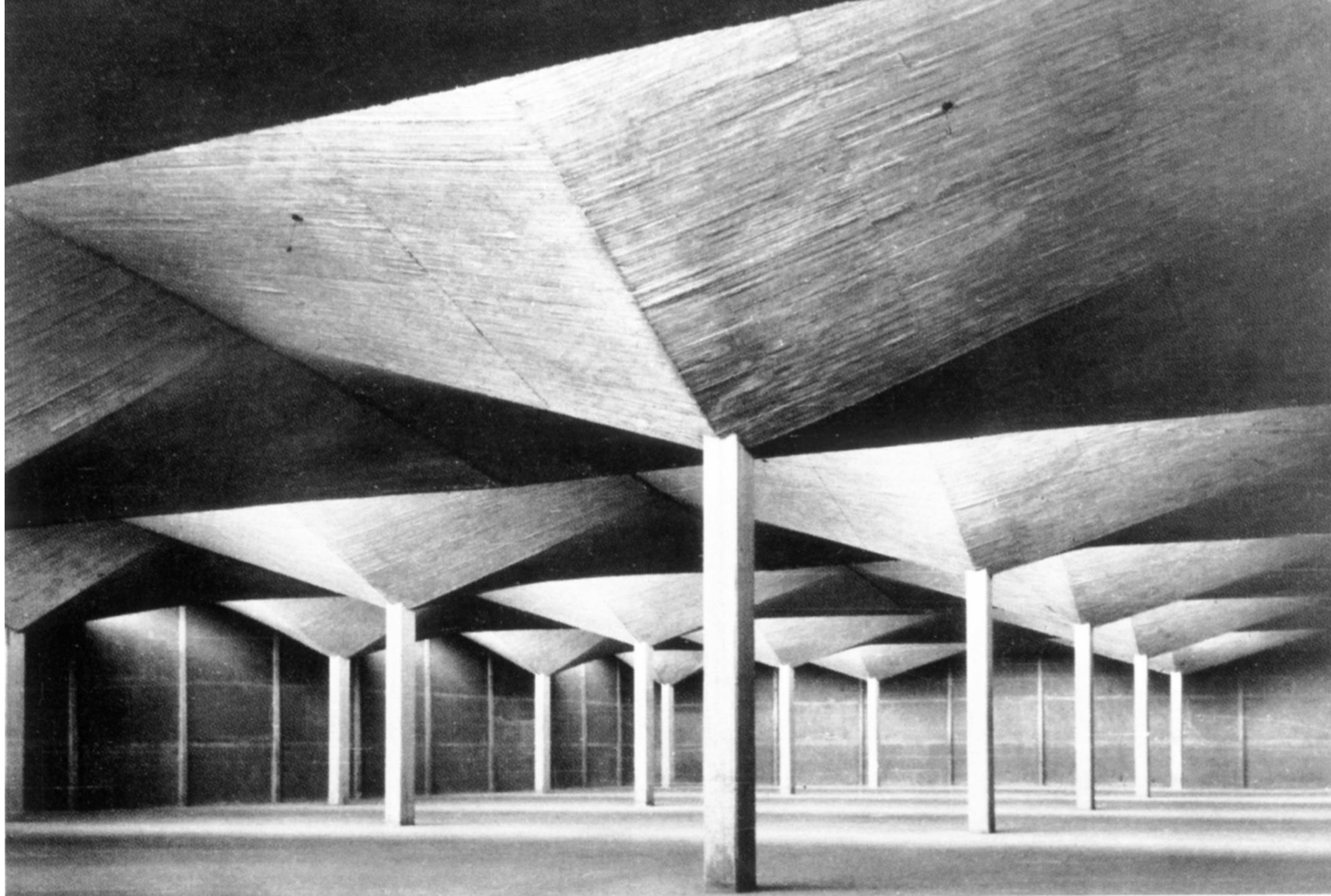
Rio's Warehouse under construction, Mexiko, Felix Candela, 1954
