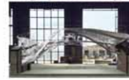
2019: Metal 3D-printed bridge (MX3D, Arup)
