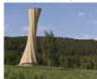
2019: Urbach Tower (ICD/ITKE)
