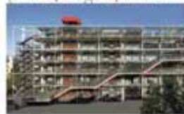
1977: Centre Pompidou (Piano, Rogers, Franchini)
