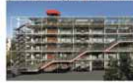
1977: Centre Pompidou (Piano, Rogers, Franchini)
