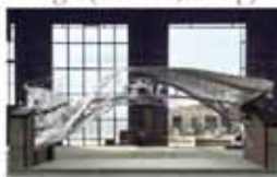
2019: Metal 3D-printed bridge (MX3D, Arup)
