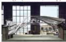
2019: Metal 3D-printed bridge (MX3D, Arup)
