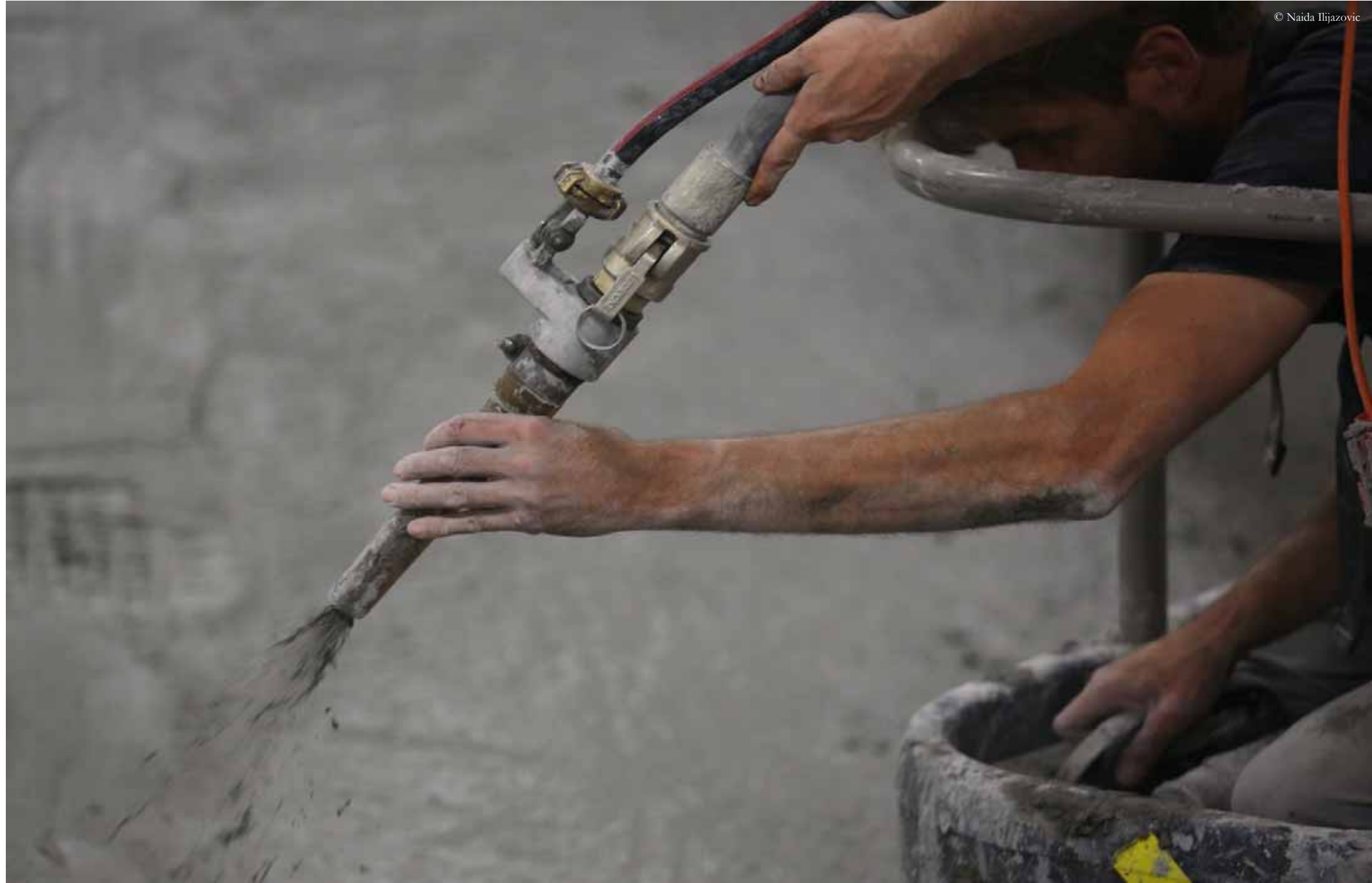
Shotcrete (HiLo, 2017, Block Research Group)
