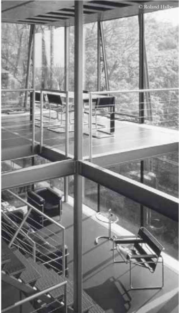
Vertical loads on the central column
