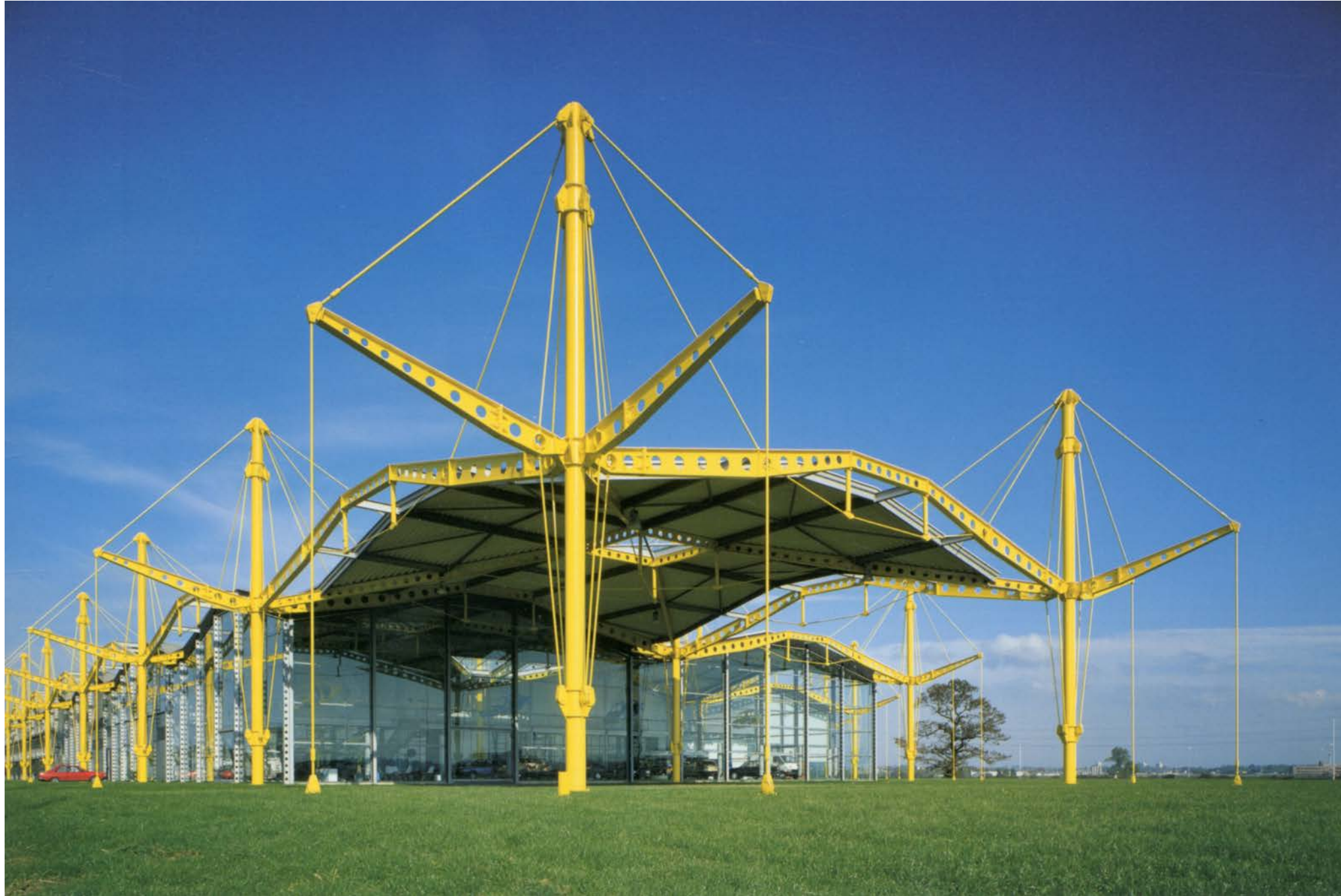
Foster+Partners: Renault Distribution Center, Swindon UK, 1983
