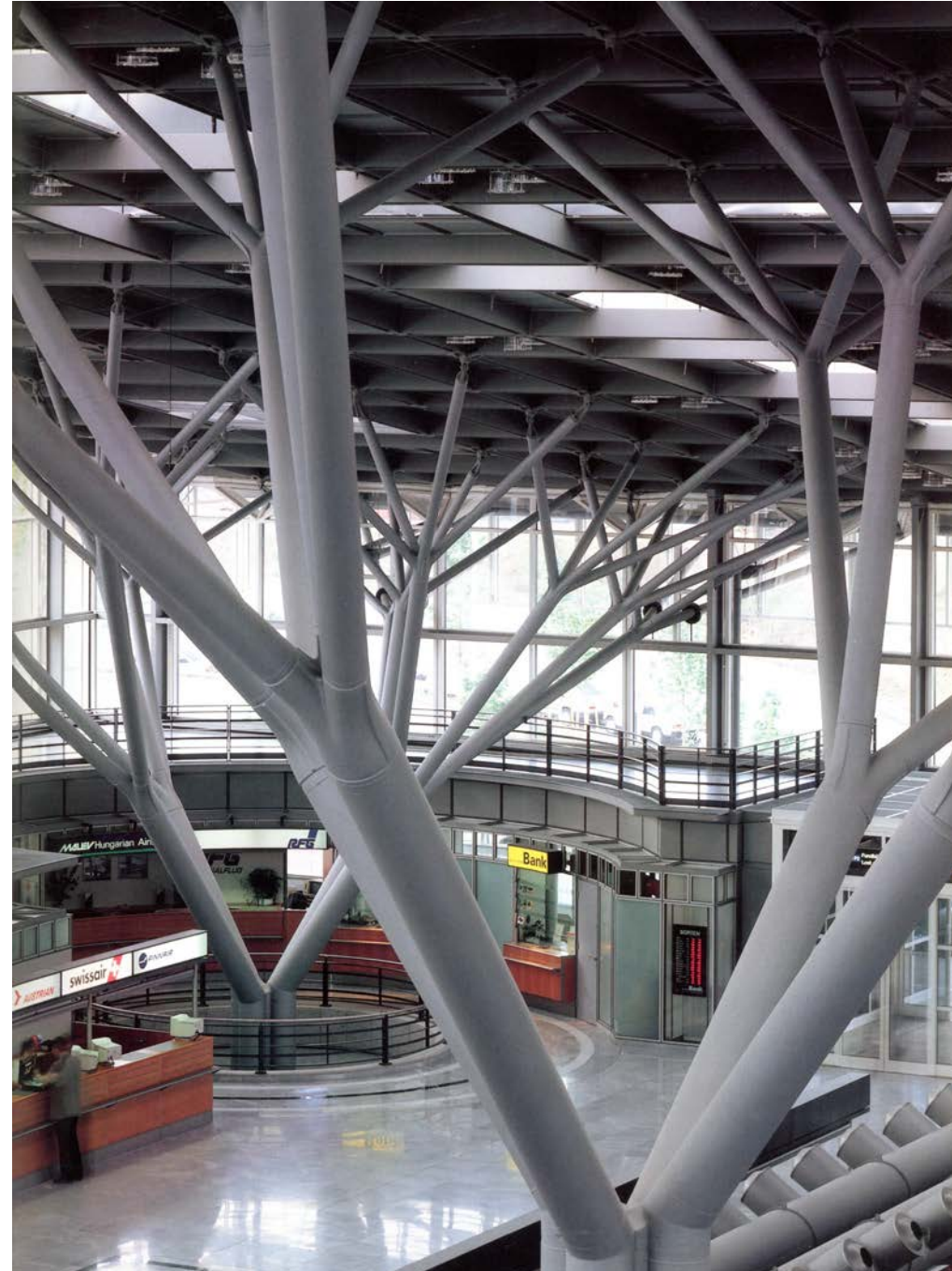
Gerkan, Mark & Partner, Schlaich Bergemann: Stuttgart Airport Terminal 3, 2004
