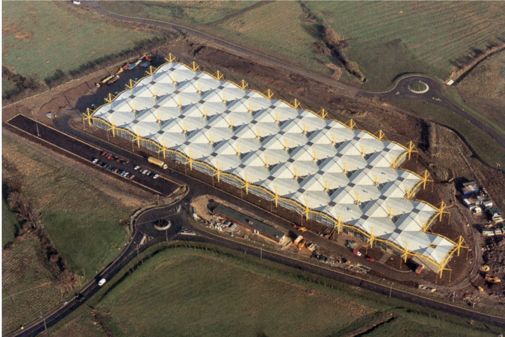
Foster+Partners: Renault Distribution Center, Swindon UK, 1983
