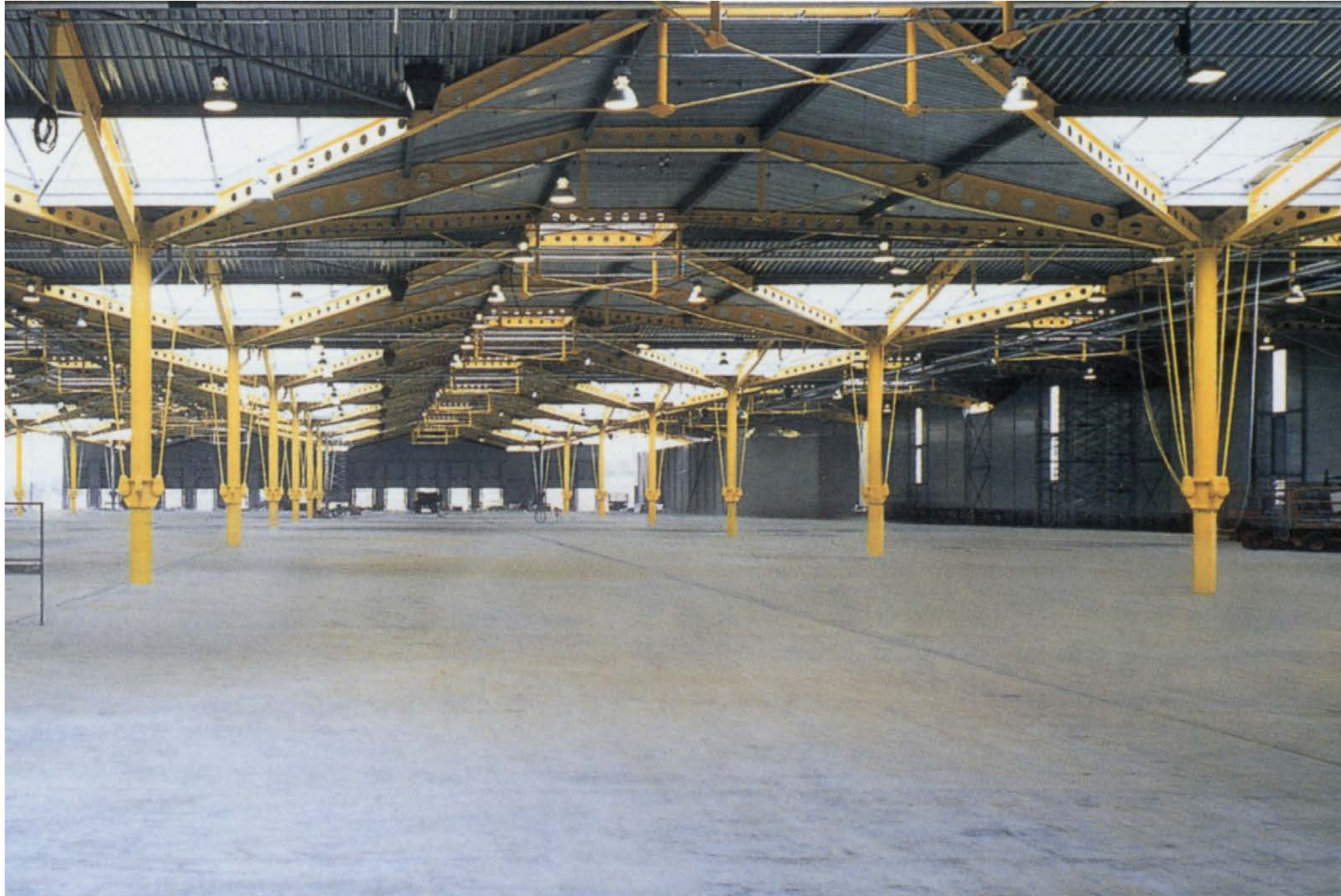
Foster+Partners: Renault Distribution Center, Swindon UK, 1983
