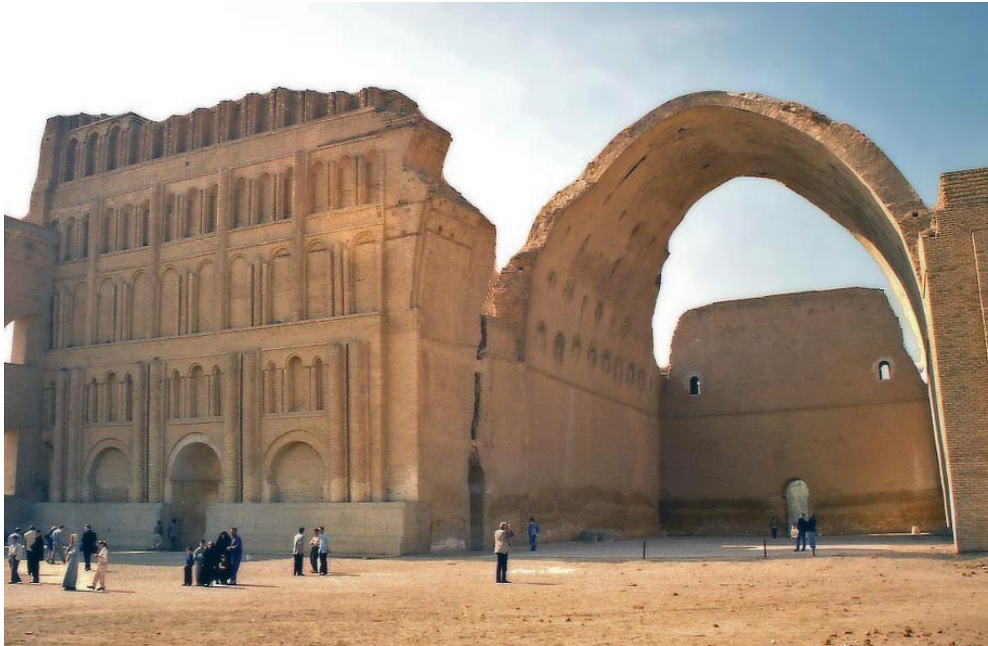
Vault to cover the courtroom in the palace of Ctesiphonte (Bagdad), III-VI-century A.D.
