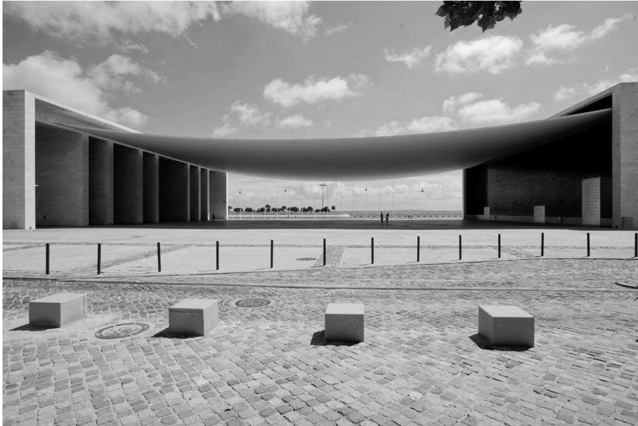
Alvaro Siza, Cecil Balmond: Expo Pavillion of Portugal, Lisbon, 1998
