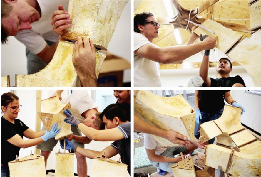
Figure 9.11: On-site assembly of the MycoTree.
