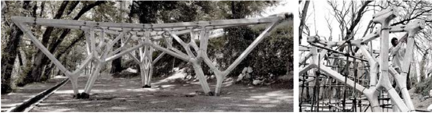
Figure 2.15: Hedracrete, first full-scale prototype designed using 3D graphic statics (Bolhassani et al., 2018).
