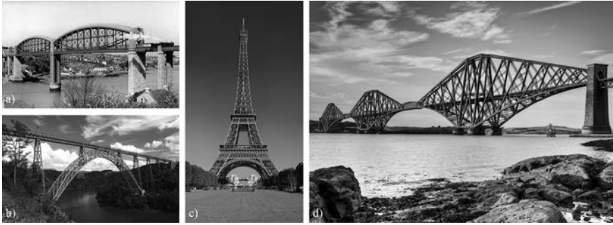
Figure 2.2: Notable cast-iron structure built in the late 19 th century: a) Royal Albert Bridge by Isambard Kingdom Brunel in 1859; b) Garabit Viaduct by Gustav Eiffel and Maurice Koechlin in 1884; c) The Eiffel Tower by Eiffel and his apprentices, Maurice Koechlin and Emile Nouguier in 1887; and d) Forth Bridge by Sir John Fowler and Sir Benjamin Baker in 1890. (Image credit: a) Norman Lockett; b) rochagneux – Fotolia; c) Wiki Commons; and d) Ray Devlin)
