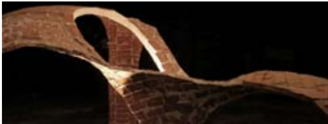
10 Final structure and TNA form finding result of the Funicular Brick Shell - 1:1 Thin-Tile Prototype.
