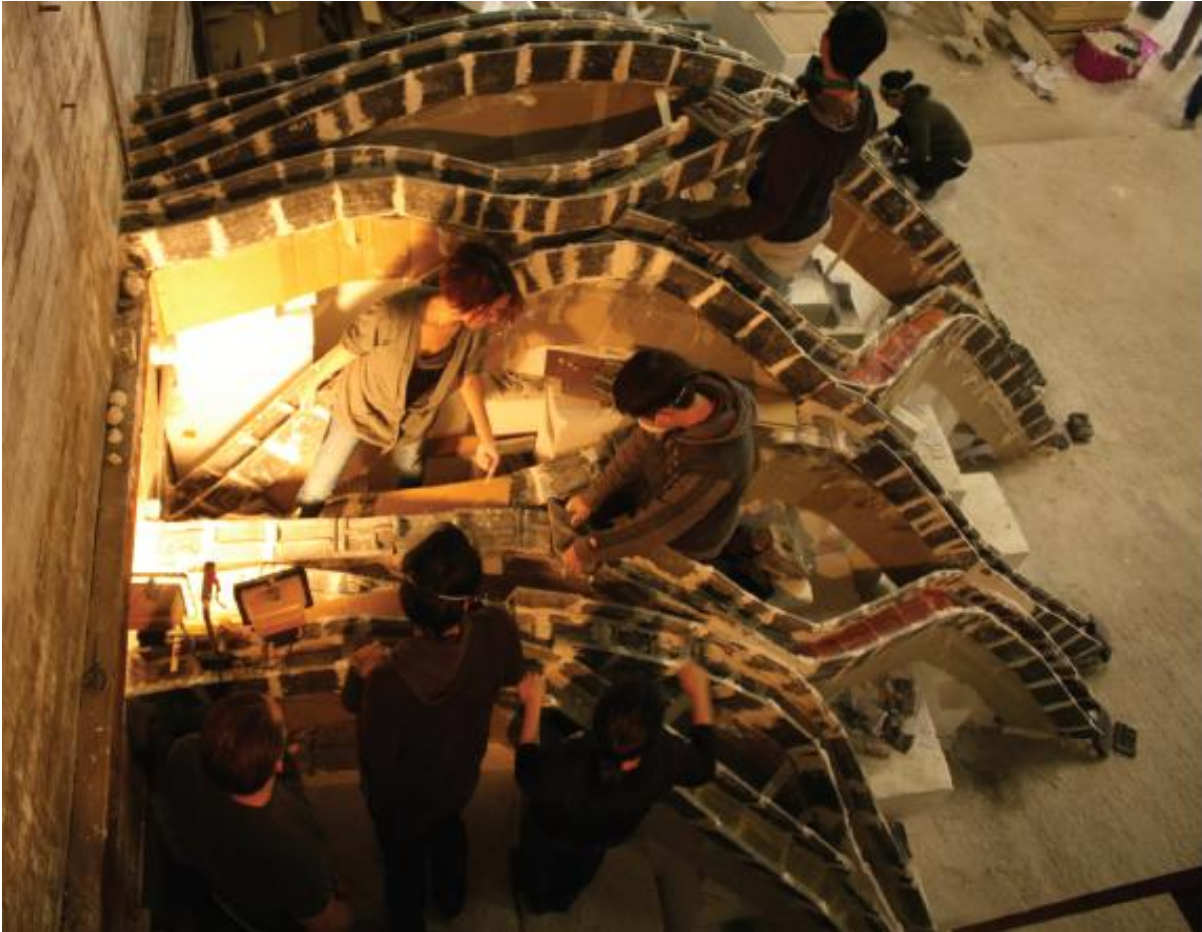
Figure 10. Aerial view of construction process for the ribs, demonstrating the laying of the tiles over the guidework. Photo: Jordan Soriot
