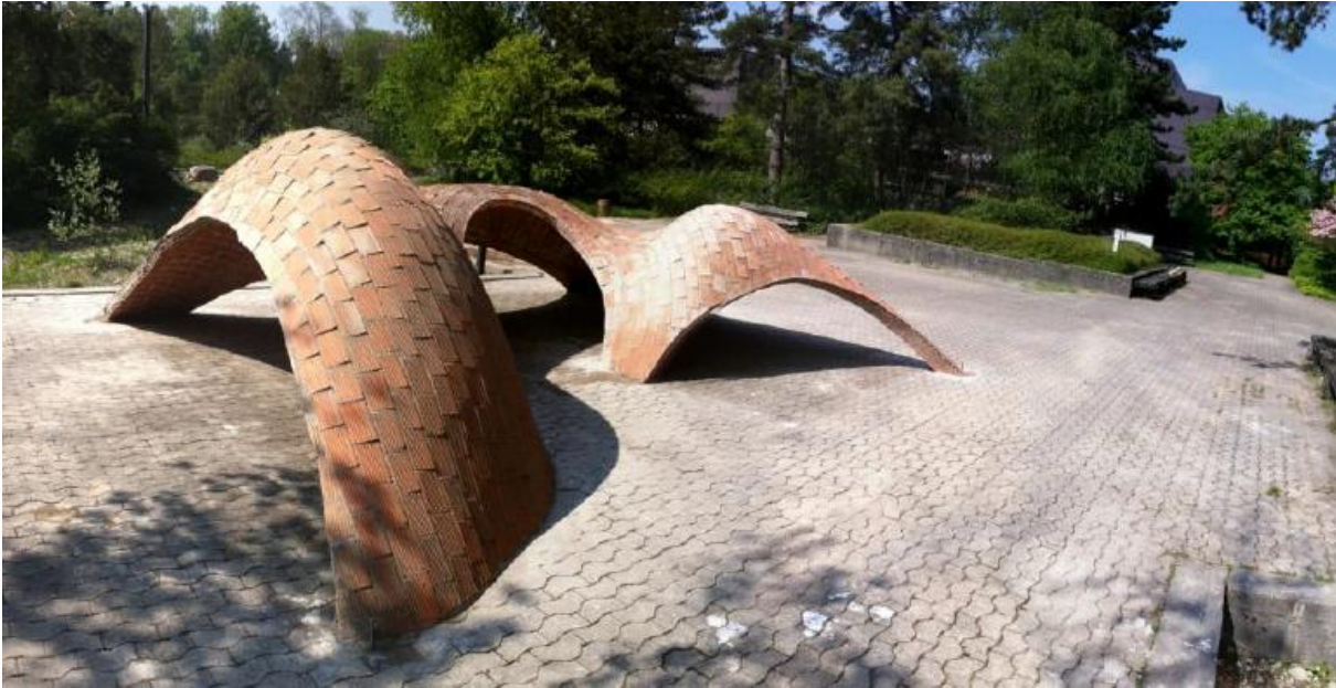
Figure 2. Freeform tiled vault built by Lara Davis (PhD research project) undertaken with the Block Research Group, ETHZ, 2011. Photo: Lara Davis.
