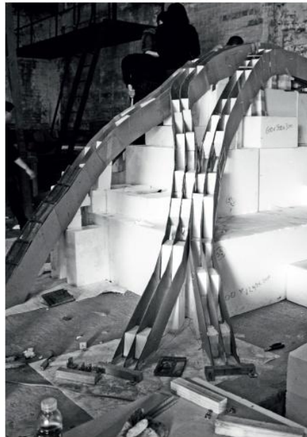
Figure 8. As the mortaring materials and method required a high level of efficiency, the construction management methods were also tested and refined to suit the build process. This included a rigorous tile cutting, numbering and stacking system, with one team mixing mortar whilst another placed and mortared the tiles. Photos: Sandra Mendonca and Natalie Ma
