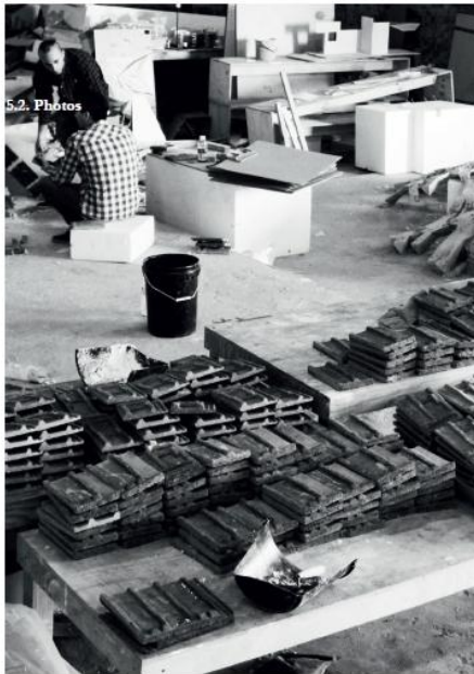
Figure 8. As the mortaring materials and method required a high level of efficiency, the construction management methods were also tested and refined to suit the build process. This included a rigorous tile cutting, numbering and stacking system, with one team mixing mortar whilst another placed and mortared the tiles. Photos: Sandra Mendonca and Natalie Ma
