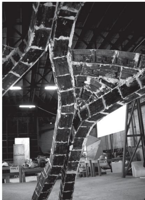
Figure 9. Rib construction and reinforcement / bracing details were developed and refined during the prototyping process that occurred concurrent to the vault building. Image shows commencement of the ‘patching’ or ‘infill’ to the ribs. Image: Masterclass students, Photo: Aaron Yeoh
