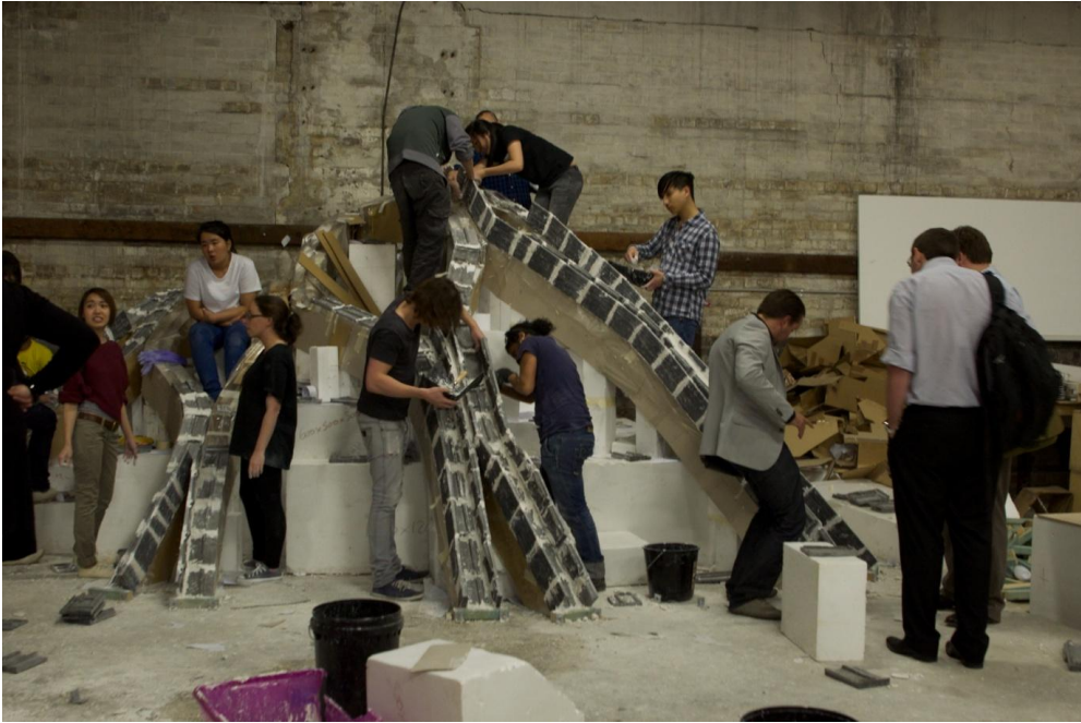
Figure 7. The vault in progress – by commencing the construction of each of the eight individual ribs at the start of the build process, an ongoing prototyping process was allowed to take place, with some demolition and rebuilding of the ribs occurring early in the build process after the geometries of several specific ribs revealed a range of construction challenges. Photo: Michael Ford_studio
