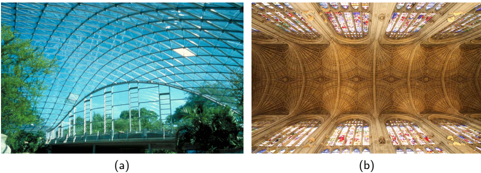
Figure 1: Two examples of structural patterns for shell-like structures: (a) beam grid of the Hippo House in Berlin, Germany (photo credit: sbp.de) and (b) voussoir tessellation of the King's College Chapel in Cambridge, England (photo credit: kings.cam.ac.uk).
