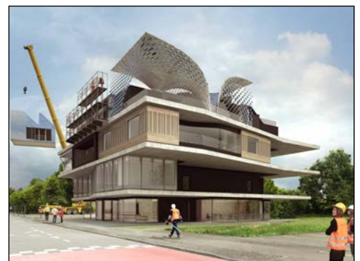
HiLo constructed on top of the NEST backbone. (image credit: Empa / Gramazio & Kohler)
